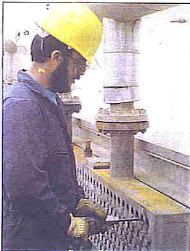
Tube ends are trimmed flush.
