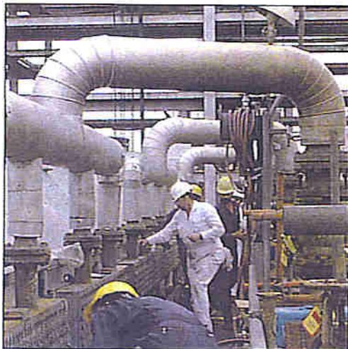
An overview of the operation in progress.
