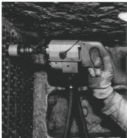
Inserts being mechanically expanded into tube ends.
