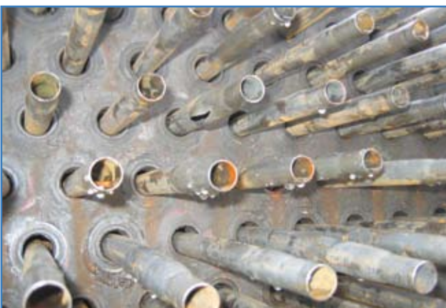
Figure 5. Post expansion of liners shown extending through header box.
