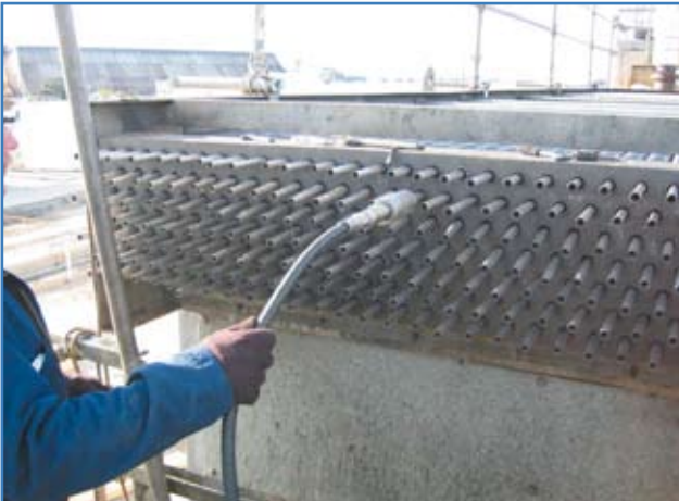
Figure 3. Inlet feed chuck for hydraulic expansion of liners to 7500 psi.
