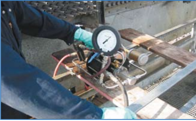
Figure 2. Portable hydraulic liner expansion pump.
