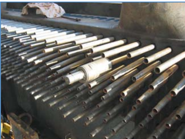
Figure 4. Outlet air bleed liner expansion chuck.
